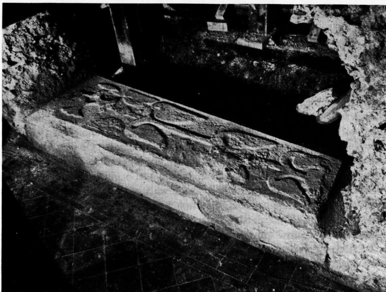
(3) East Shefford Church: Caen stone coffin recently found in the thickness of the chancel's north wall.
